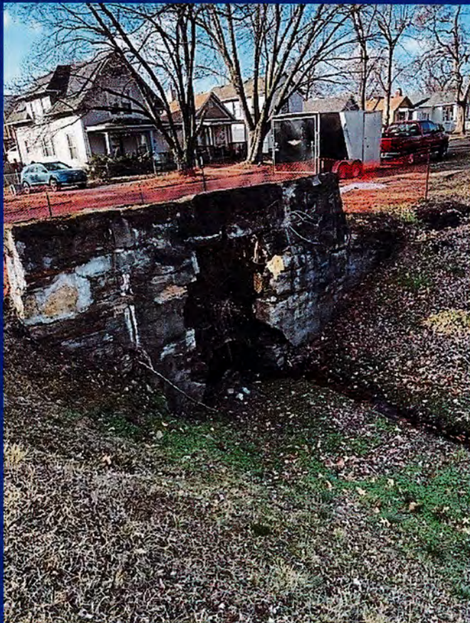
38 FAILED HEADWALL
