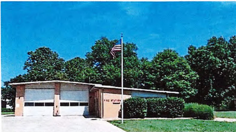
Fire Station #3 was built in 1965. At the time, ADA and separate gender facilities were not considered. Additionally, the facility continues to experience drainage and sewer problems.
