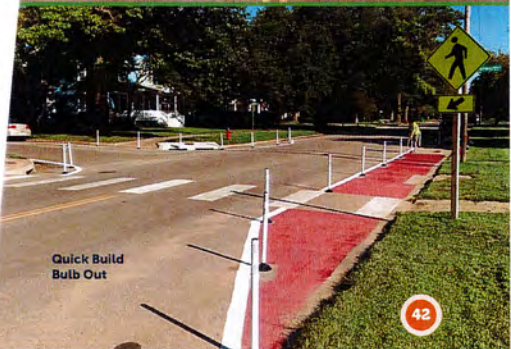
Quick Build Midblock Crossing Bulb Out
